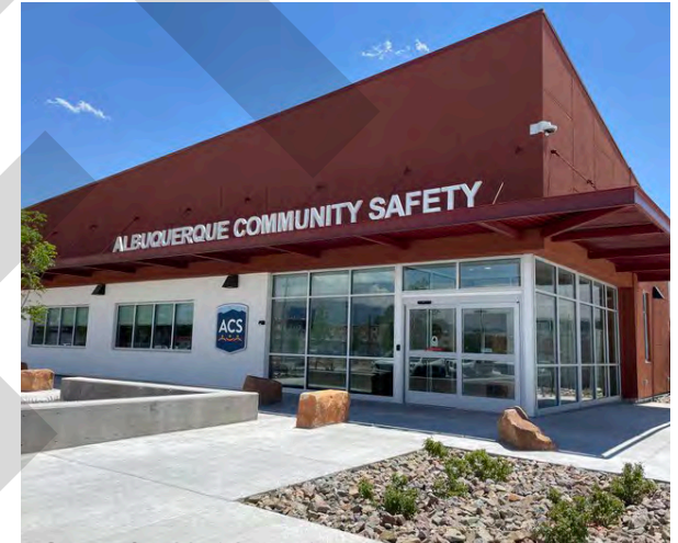
FIGURE 60. ACS at San Mateo Blvd
