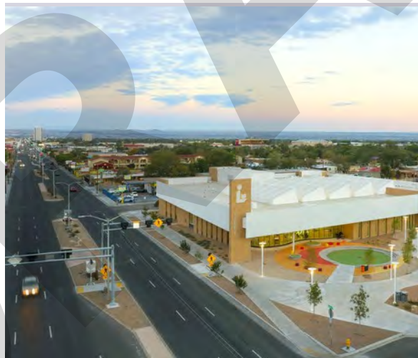
FIGURE 91. International District Library
