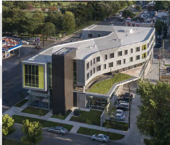
FIGURE 140. Northtown Apartments and Library, Chicago, IL
