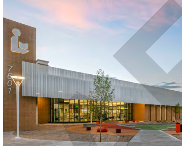
FIGURE 6. CABQ International Library (Source: RNKM Architecture)
